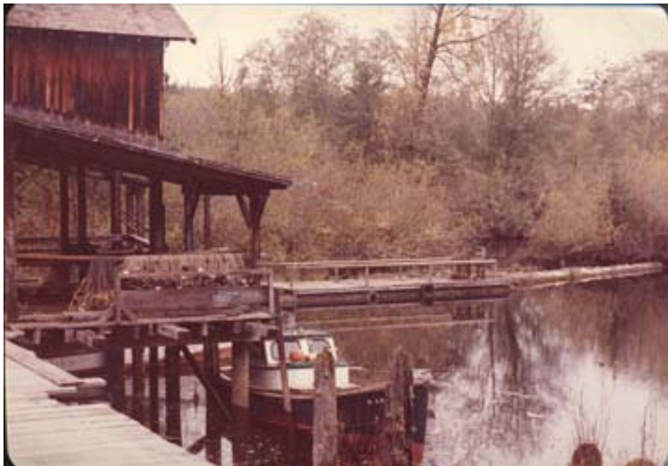
The Brownsmead warehouse near Davis Bottom Road
